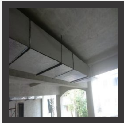
Duct with Nitrile Rubber Insulation
